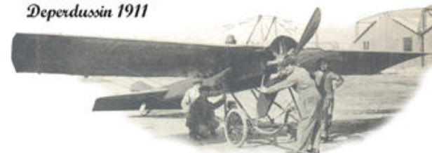
Gnome 50 HP engine, two bladed wooden propeller made by Paulin Ratier.
